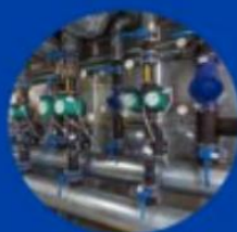
Boiler/ Mechanical Rooms
